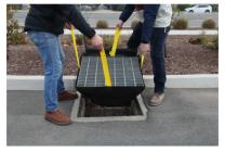
**2.** Using the straps, lift the grate and place it back in the storm drain with the YJ underneath. If there is a curb inlet, make sure the foam backer is on the side of the curb inlet. Remove the foam backer if there is no curb inlet.
