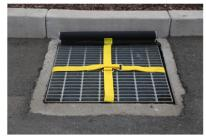
**Alternate Steps 3 & 4.** Once the filter is put in place, take a carabiner from one one strap and attach it to the loop on the other end of that same strap. Repeat for the other strap.
