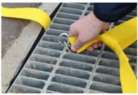
**4.** Pull the carabiner side through until the strap is tight and attach the carabiner to the grate. Repeat steps 3 and 4 for the other high visibility strap.
