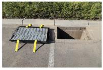
**1.** Remove the YJ from the package. On a flat surface adjacent to the drain, remove the grate and place it on top of the YJ (with straps facing up). Ensure all four of the filter edges are visible around the edges of the grate.
