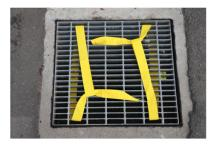
**5.** The Hornet's Nest Drain inlet filter is now successfully installed.
