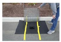
**1.** Remove the drain grate and unfold the Hornet's Nest and place it centered and into the storm drain you wish to protect. Make sure the high visibility straps are facing up.
