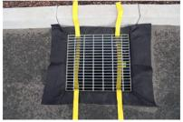
**2.** Place the grate back into the storm drain and while doing so, pull each of the four ends of the high visibility straps up through the grate openings.
