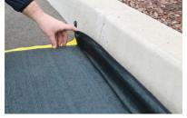
2. Each long side (front and back) of the AGF has a rigid slat that can be lifted vertically and pressed against the curb to provide protection to a curb inlet. If there is not a curb inlet, simple leave the AGF flat over the entire grate.
