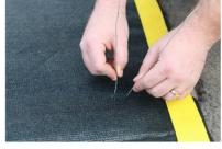
**4.** Pierce the AGF with both ends of the baling wire through the bottom of the filter and feed upward through the unit so the baling wire is exposed at the top.
