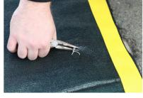
**5.** Secure the filter to the grate by twisting the baling wire. Once twisted, trim the excess wire and flatten it to hide sharp edges. Repeat steps 3-5 for the remaining corners
