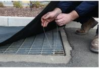
**3.** Starting with one corner, lift the filter to expose the grate and loop the baling wire down and around one of the grate pieces.
